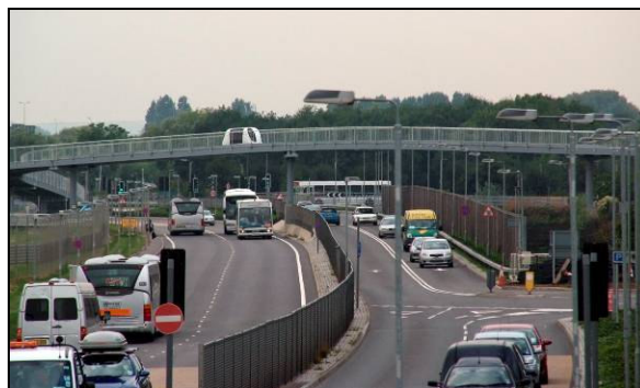
Figure 1.8: High-visual-impact safety rail (LHR) is not appropriate
