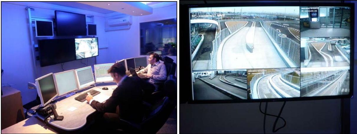
Figure 1.20: Heathrow OMF control room & control room CCTV
